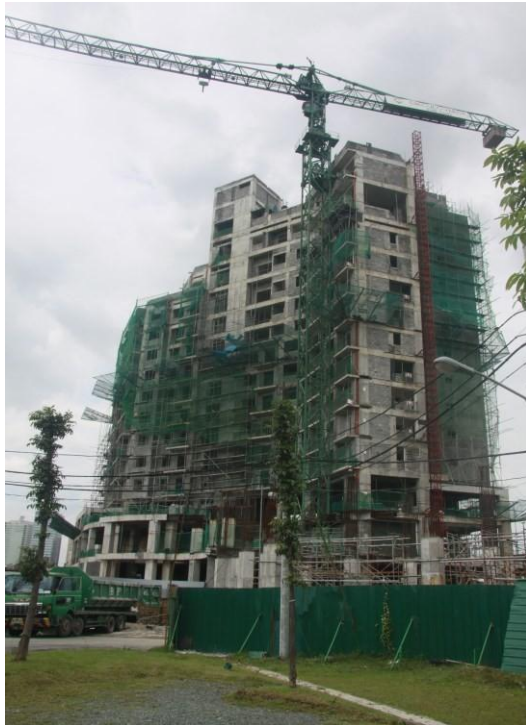
CIRKULO VERDE PASIG CHB LAYING & PLASTERING WORKS
