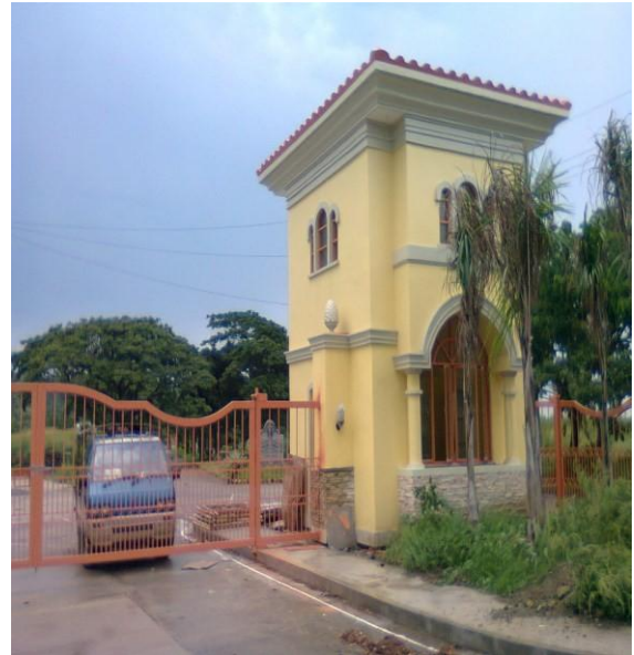
Valle Verde South, Biñan Laguna Guard House and Gate
